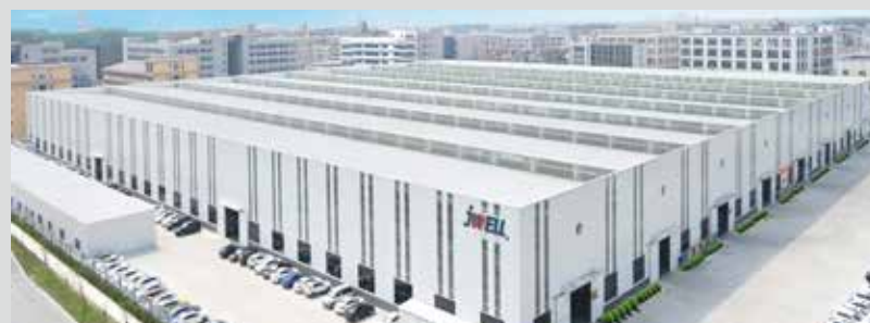
Jwell Machinery Haining Factory 金纬机械海宁厂区
